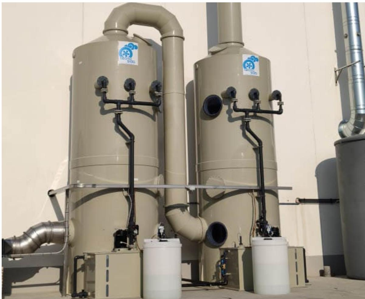
The gas flow full of water goes through a droplet separator before being carried in the second scrubber. This one allows the acidic substances to be reduced before the emission in the atmosphere. For this reason, it has a tank for the soda (base reagent) which is added to water. The solution designed and created by Tecnosida® has allowed the acidic and base gases to be reduced, therefore solving the client's problem and reducing the emission within the limits established by Law.
