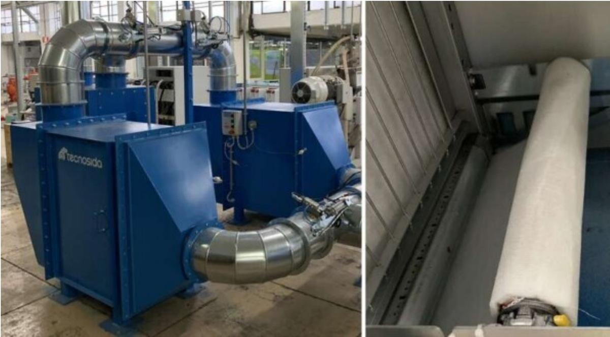
After this pre-filtering phase, the air flow is carried by the process fan into the THEROX regenerative thermal oxidizer. The RTO designed for this application consists of:
