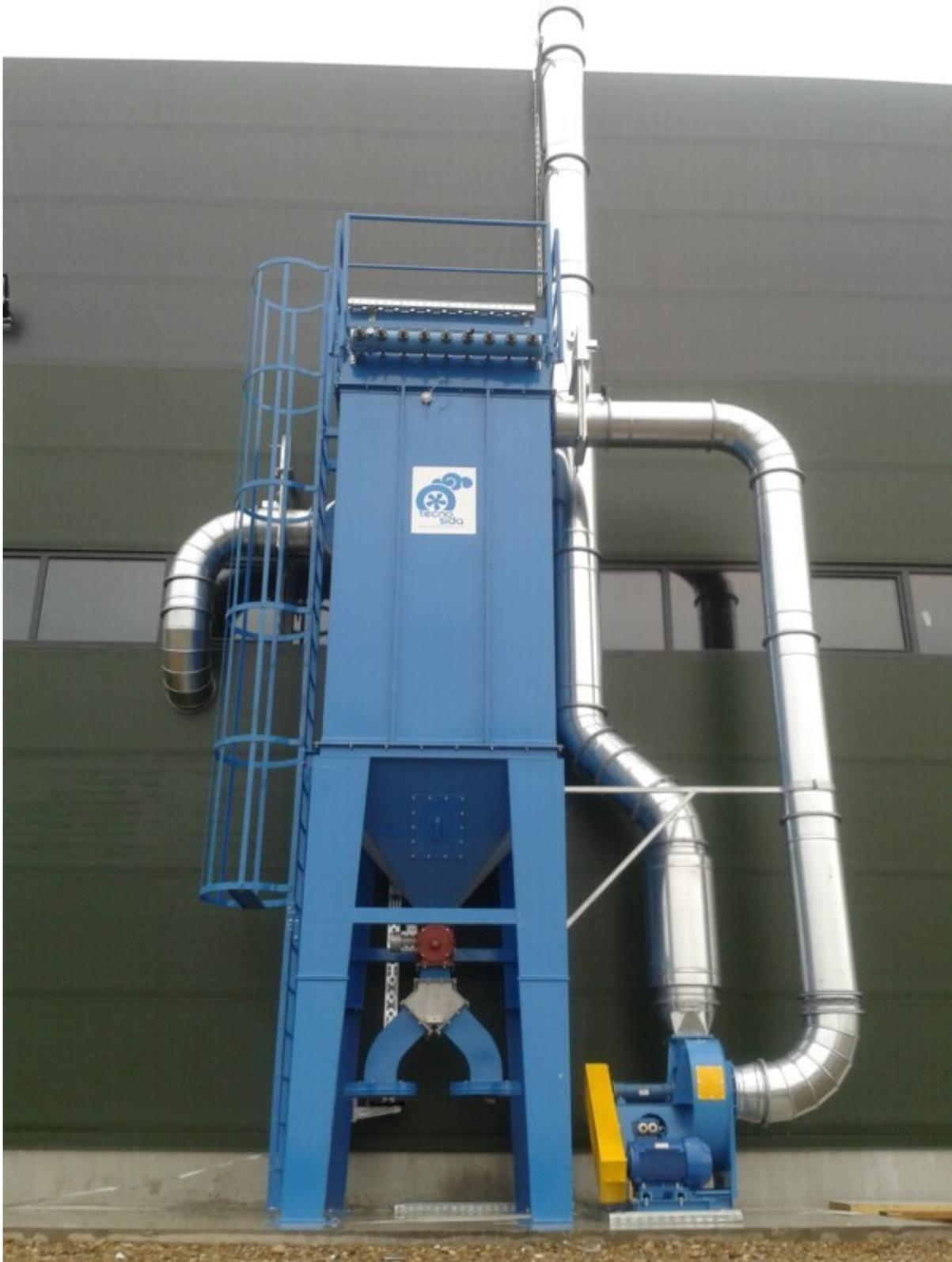
All dust sucked by these systems is then conveyed to a Dustdown bag filter where the airflow is treated and then, once purified, it is released into the atmosphere.
