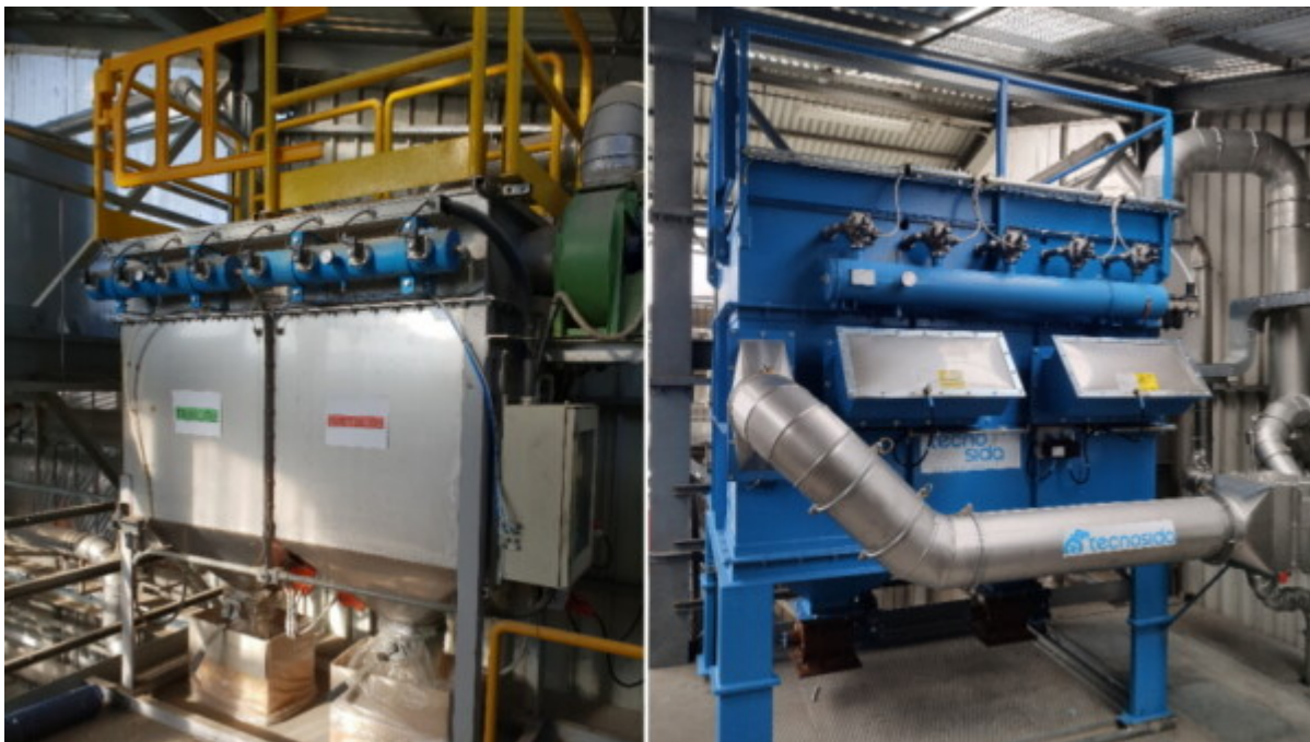
ATEX bag filter for insecticide powders
